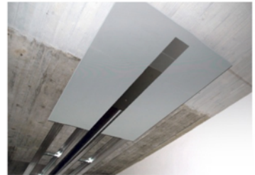
Radiant cooling panels
